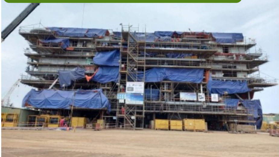
Topside and jacket foundation for HL2 and HL3 offshore substations progressing as per schedule.
